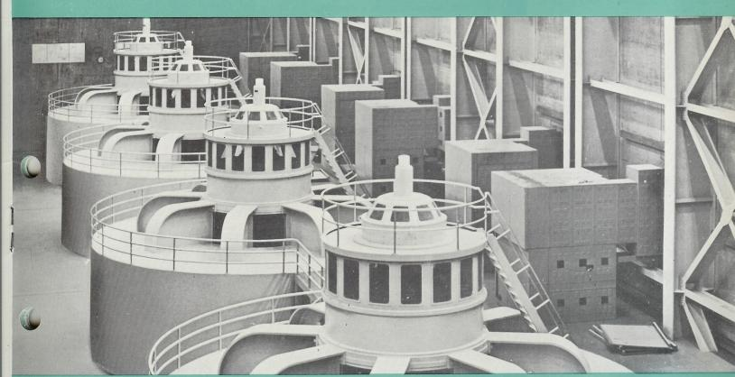
Four generators rated 75,000-kva, 180-rpm at U.S. Bureau of Reclamation, Hungry Horse Dam, Coram, Montana.
