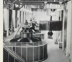
5 G-E generators, each rated 82,500-kva, 180-rpm in Nevada wing of Hoover Power Plant
