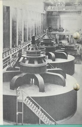
Two of five 75,000-kva, 138-rpm generators in the Shasta Power Plant, Central Valley Project, California.
